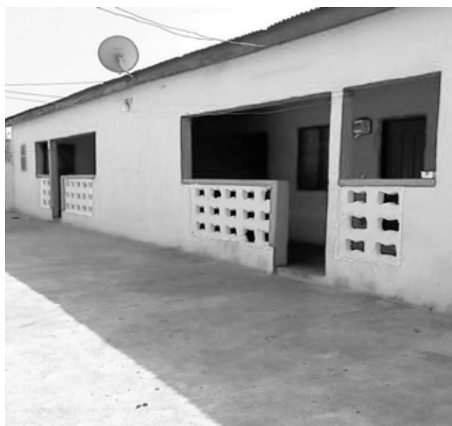
Nambiri Primary School - before (top), after (above)
