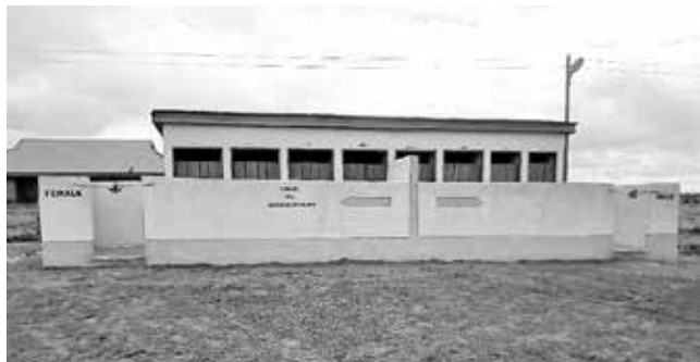
New toilet block, Walewale Vocational School
