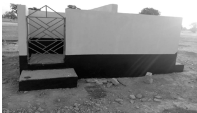
Zuarungu Moshie JHS - newly rebuilt urinals
