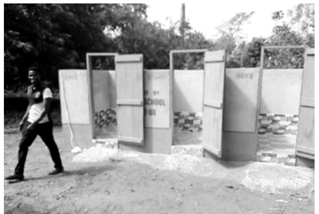
New toilet block, Manyiha No.1 Basic School
